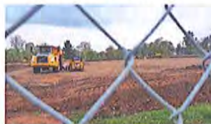
NORA G. HERTEL/USA TODAY NETWORK-WISCONSIN Construction of the Timberwolf Suites, shown on May 16, is underway near the Northcentral Technical College campus. It's geared toward students.
