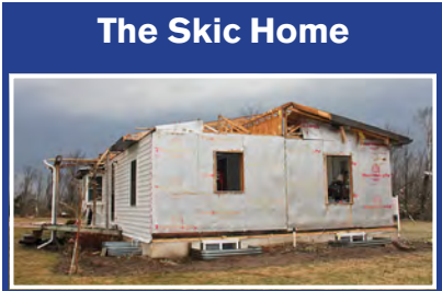
Rose Skic's home on Hwy. K is a total loss, although some of the home's contents were saved. Rose Skic photos
