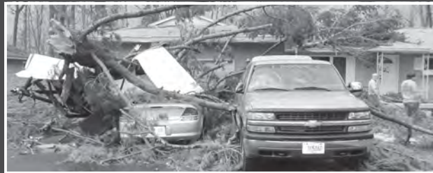
Falling and flying trees and limbs did the most damage at the Schreiber home, including a limb that impaled itself through their roof. Teresa Schreiber
