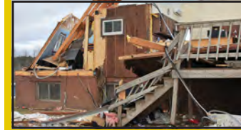
Above: The home of Lisa and Mike Handlin on Balsam Blvd. was completely destroyed. Mike Handlin
