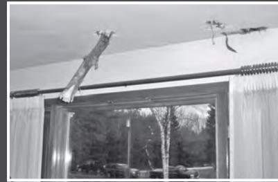
When the Schreiber family came up from the basement, they could immediately smell pine. Here pine limbs came through their roof and ceiling. Outside, pine trees are down all around the home. Teresa Schreiber
