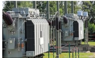
Electrical Power Distribution
