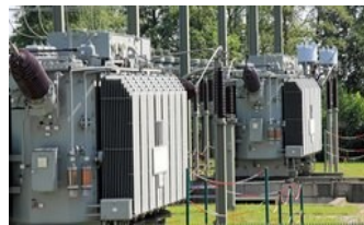
Electrical Power Distribution
