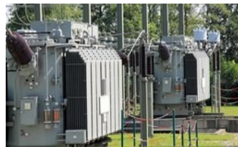
Electrical Power Distribution
